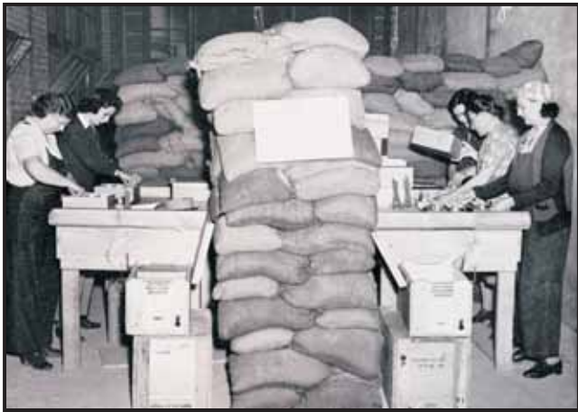
Employees tape safety blocks in fuses before shipping. The sandbag walls provide protection and a place where ammunition can be thrown in fear of detonation.
