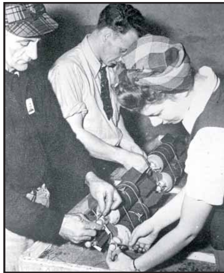
Employees tape safety blocks in fuses before shipping. The sandbag walls provide protection and a place where ammunition can be thrown in fear of detonation.
